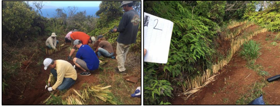
Figure 2-29. West Maui erosion control in watershed using vetiver grass to catch sedimentation. Planting vetiver rows (left); finished vetiver rows (right). Source: West Maui Ridge to Reef
