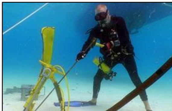
1982 1983 Figure 2-43. A diver installs a mooring buoy on the seafloor. Source: NOAA
