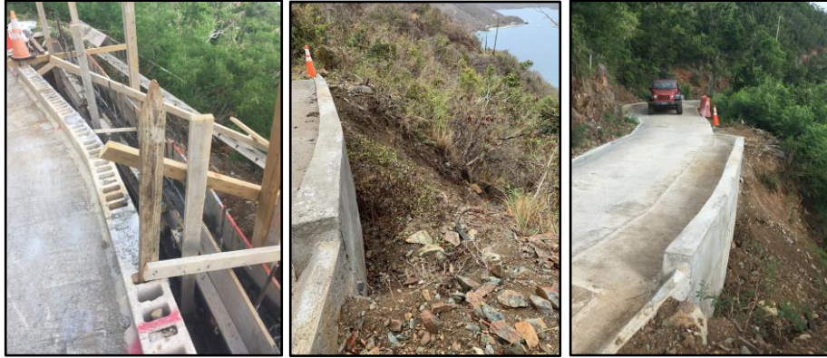
Figure 2-32. Freeman's Ground, St. Johns, USVI retaining wall for road stabilization. Source: Coral Bay Community Council
