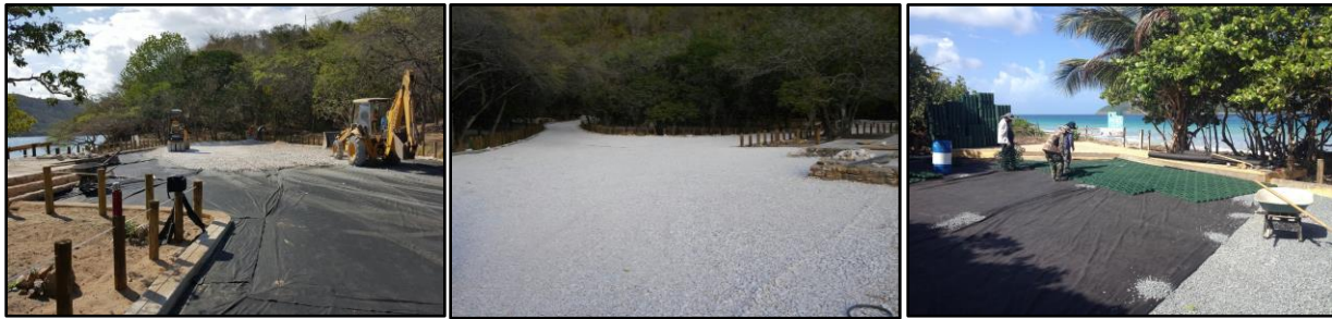
1881 1882 Figure 2-40. Examples of low impact development practices and permeable parking areas that allow for filtration of rain/run off. 1883 Source: Protectores de Cuencas
