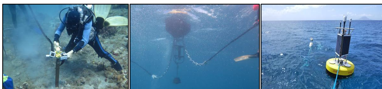
1110 Figure 2-9. CREWS buoy installation. Left: The core barrel drill; Center: Buoy before attachment underneath the water; Right: 1111 buoy above water. Source: NOAA Atlantic Oceanographic and Meteorological Laboratory 1112
